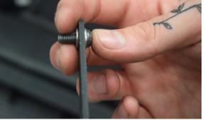
15. When installing the hard pipe support bracket, ensure the washers are positioned like this.
